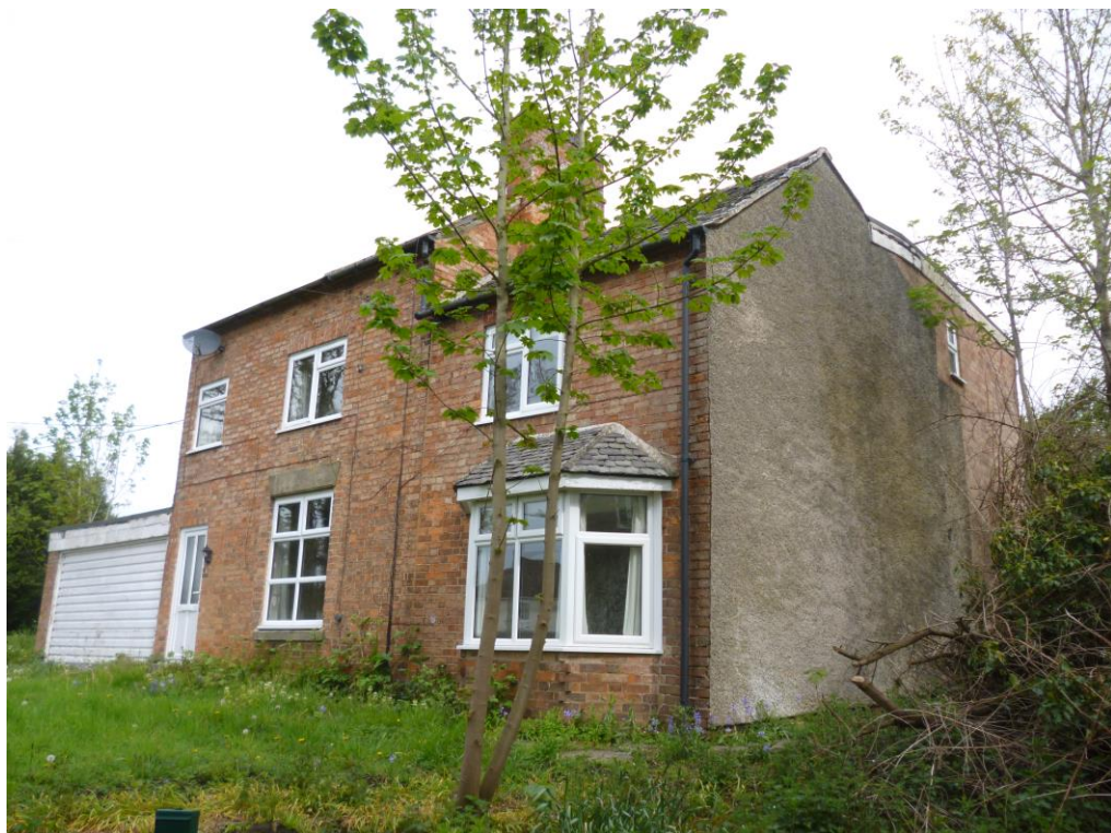
1: Scotland House – Existing dwelling at the application site
